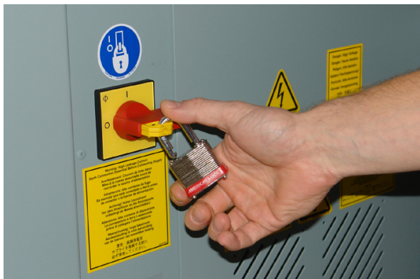
[47] AC Power Switch and Lockout
